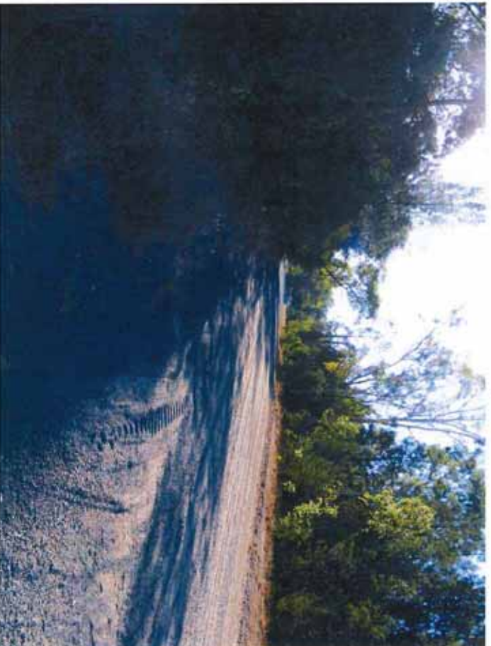
Figure 3: Gil Gil Creek Road looking south from quarry entrance
